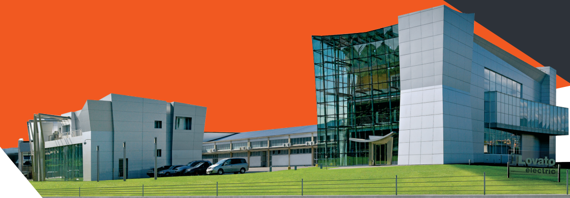
LOVATO Electric headquarters - Bergamo (ITALY)
