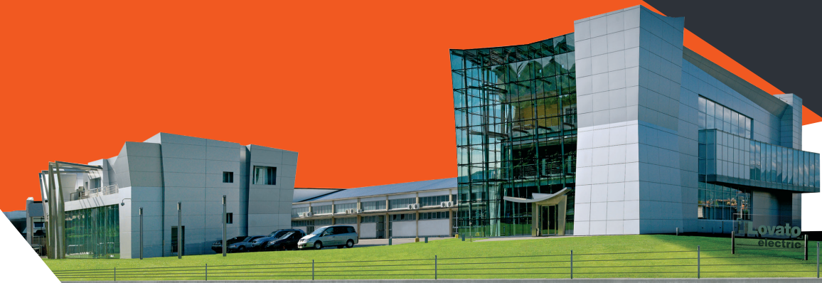
LOVATO Electric headquarters - Bergamo (ITALY)
