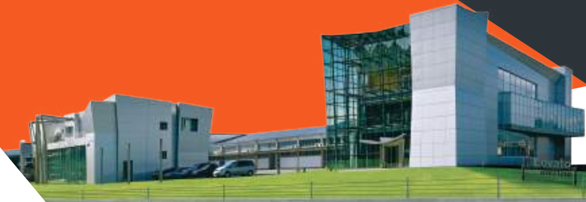
LOVATO Electric headquarter - Bergamo (ITALY)
